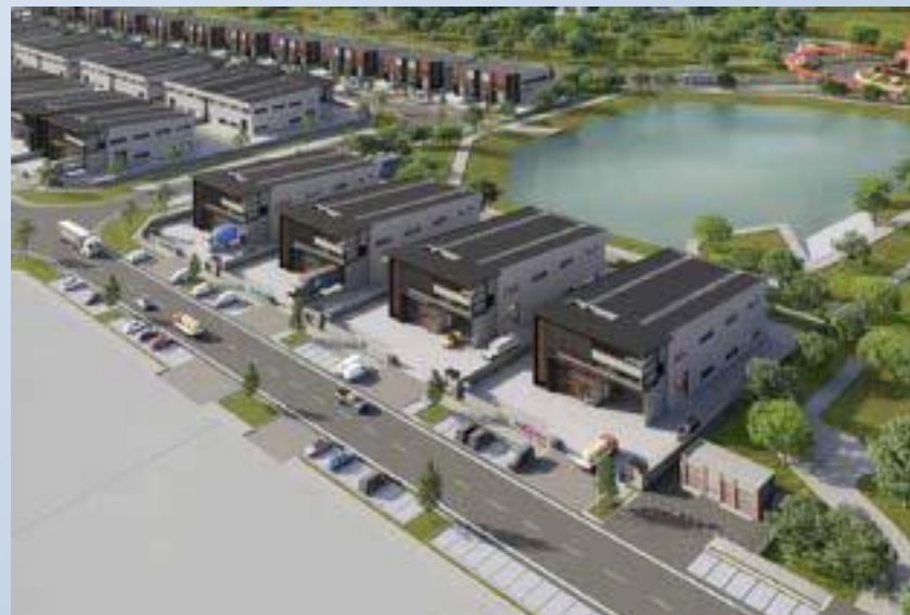
Projek Pembangunan Centralized Labour Quarters (CLQ) di Elmina Business Park
